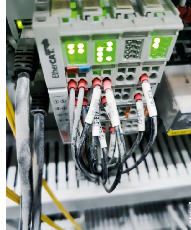
EtherCAT plays a central role in controlling the drive technology. The distributed clocks function enables system-wide synchronization of all wall panels in the installation
