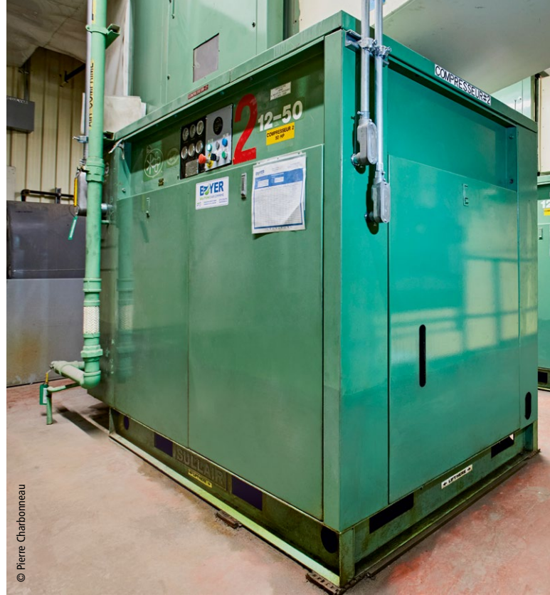
EtherCAT communication networks a wide variety of devices in the plant, including these compressors.
